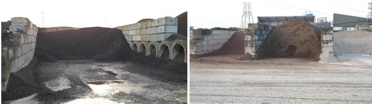
Figure 2: Bays created at Creagh to stockpile the CDW aggregates (04/10mm on the left and 0/4mm on the right).
