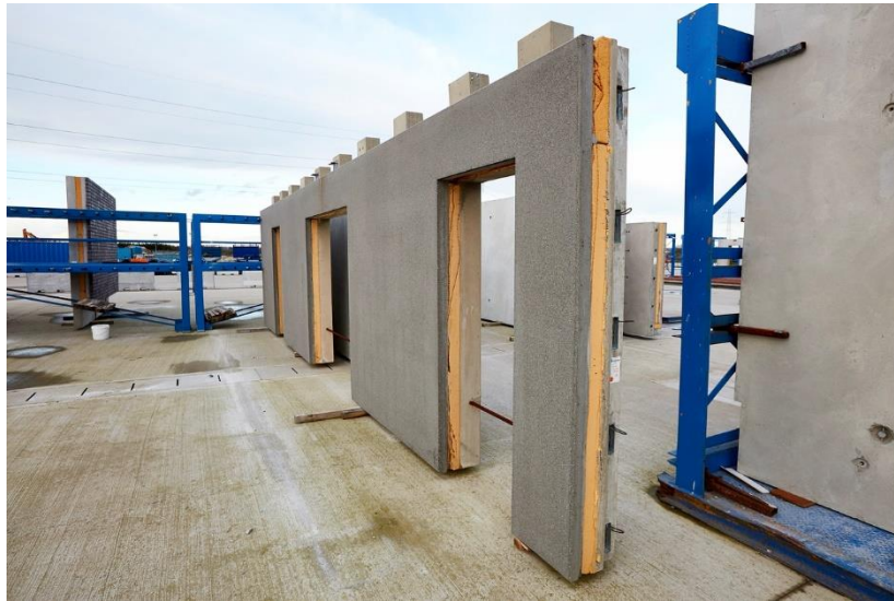
Figure 6: Picture of sandwich panel
