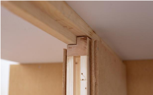
Figure 3 – Standardised elements with reversible connections at the head
