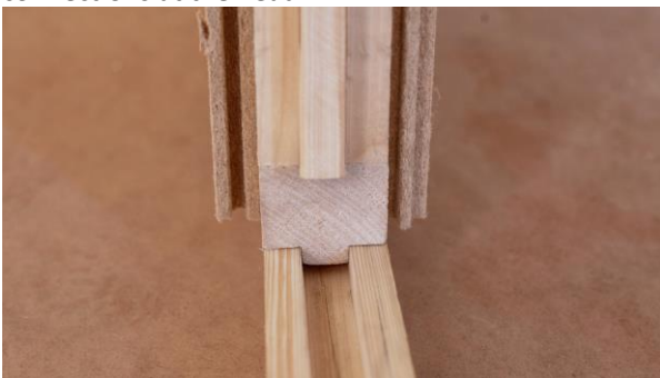
Figure 4 – Standardised elements with reversible connections at the foot
