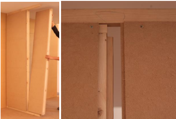
Figure 5 – Standardised elements with reversible connections between elements
