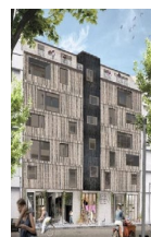
Building design for a reversible RE 4 building made out of recycled timber
