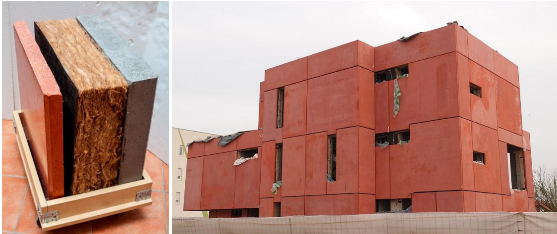
Figure 15: ECO-SANDWICH prototype and first house in Koprivnica
