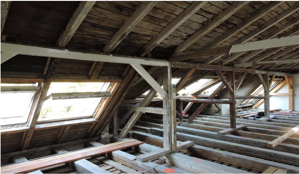
Figure 90 On-site Inspection of a roof structure.
