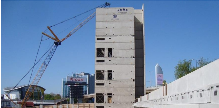
Fig. 6 (a-b): 3D Volumetric Precast Concrete Construction [161UK]
