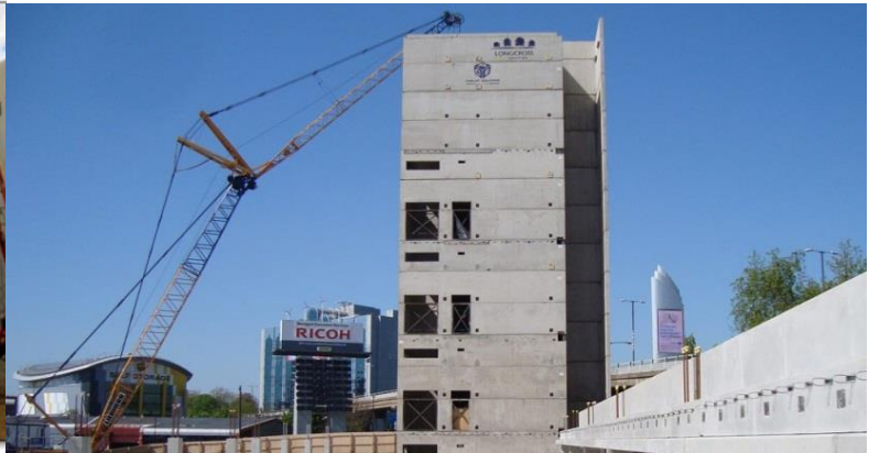
Figure 13. Construction of 20 m high modular stair and lift core
