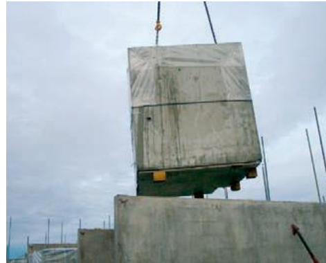
d) Stairwells are installed
