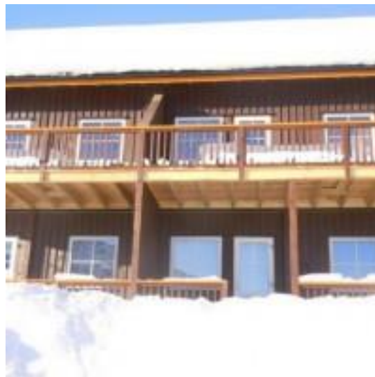
Figure 4. Example of modular house [9]
