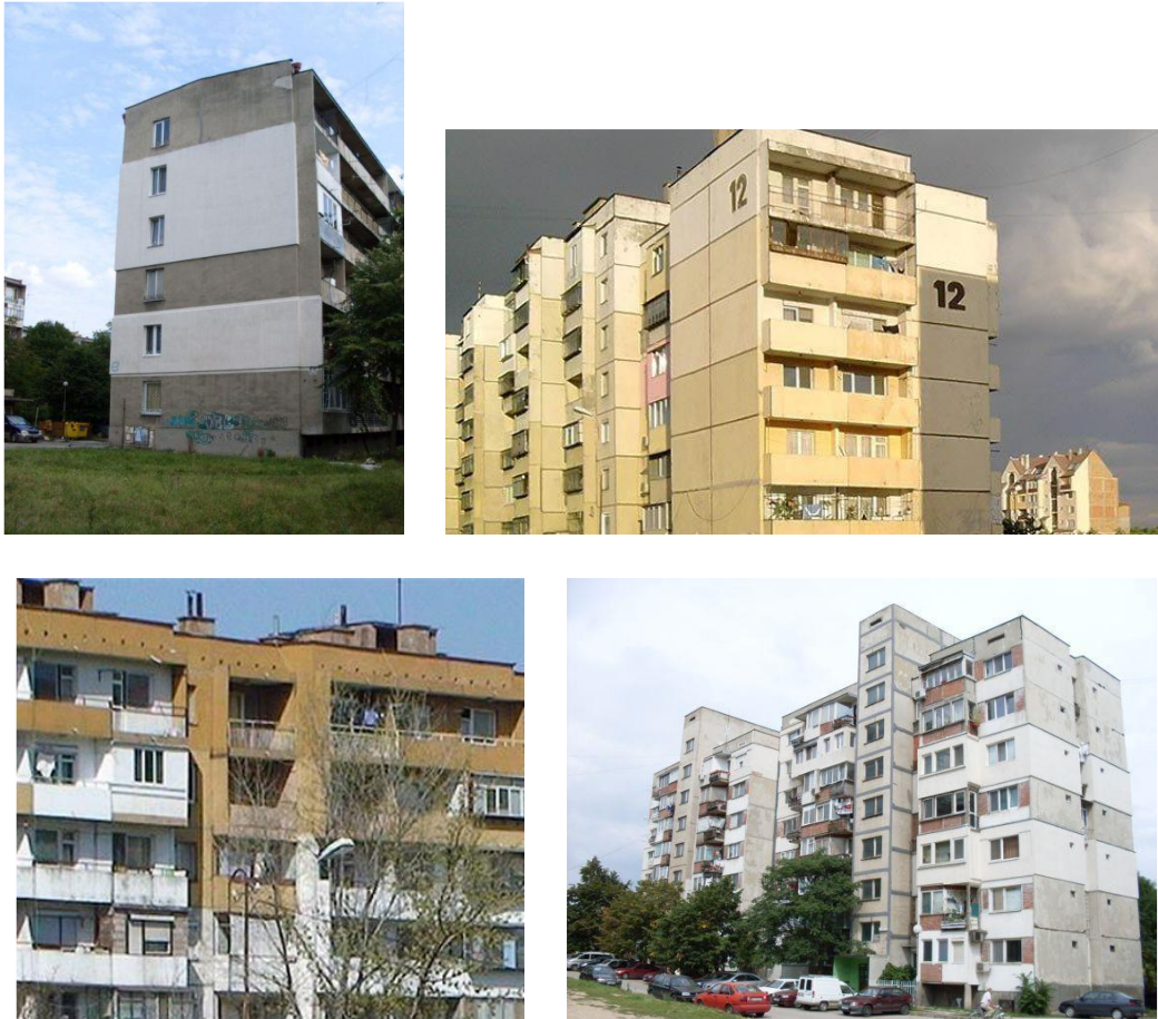
Figure 1. Experience of “large-panel system” residential buildings in Bulgarian cities [13]
