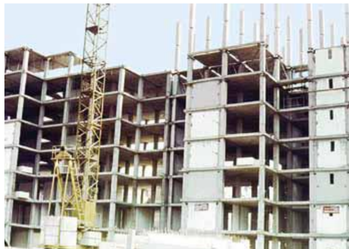
Figure 3. All-precast concrete dual structure during erection.[8]
