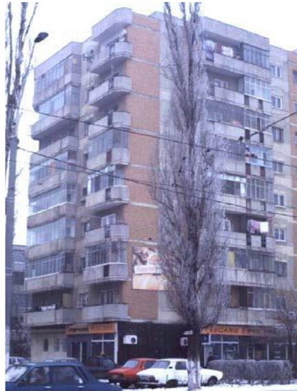
Figure 2. Typically precast concrete panel apartment building in Romania.[7]
