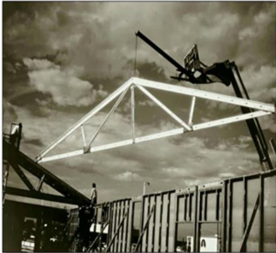
Figure 8. Installing roof trusses
