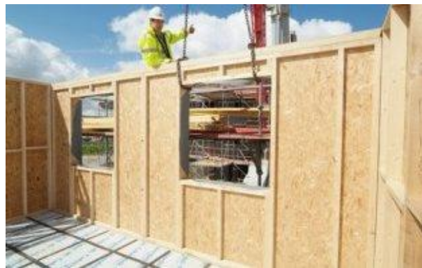
Fig. 8: Installation of Open Panel Timber Frame [164UK]
