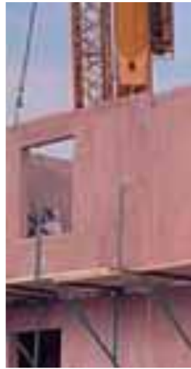
Figure 2. Prefabricated panels made of concretes made with recycled aggregate produced from mixed CDW [13]
