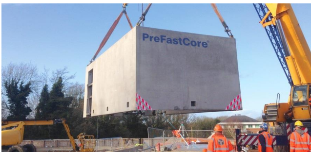
a) Installation of a precast concrete modular unit
