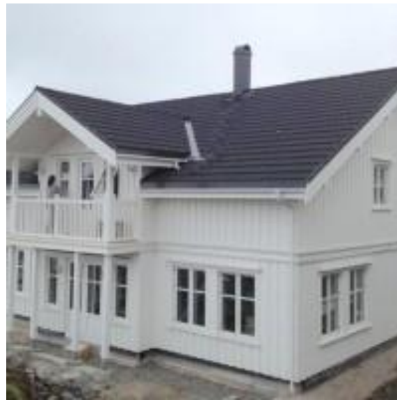
Figure 3. Example of panel house [8]
