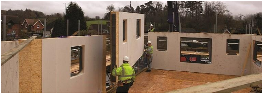
Fig. 7: Installation of SIPS [163UK]
