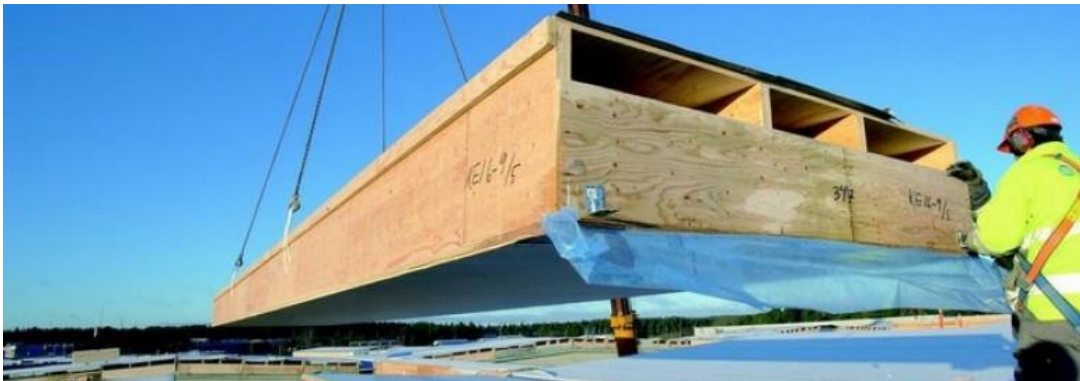
Fig. 10: Installation of prefabricated Floor panel [167UK]
