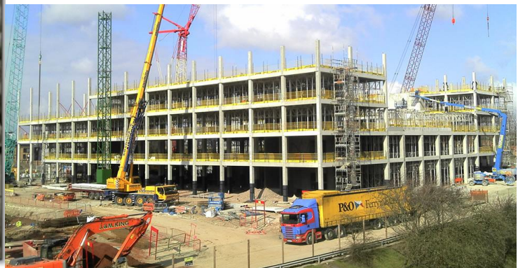
Figure 9. Precast concrete beams and columns [66]
