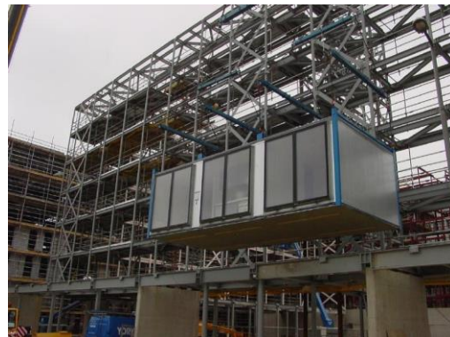
h) Installation of a module on a steel podium
