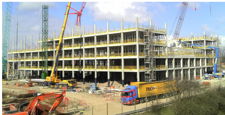
Fig. 1: Precast concrete beams and columns [155UK]
