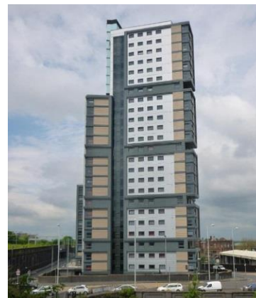
Fig. 5: (a-l): Modular Construction using light steel framing [159UK]
